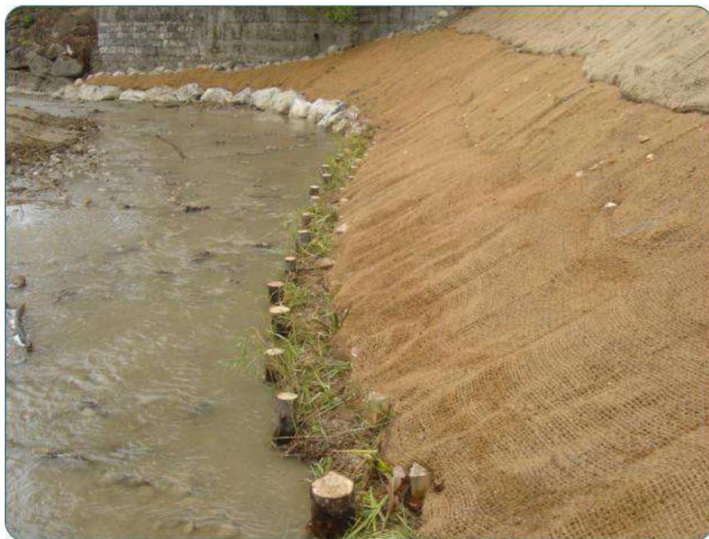
**EXEMPLE DE MISE EN ŒUVRE DE TOILE COCO AVEC AGRAPHE BOIS ET DE FASCINES D'HELOPHYTES (SOURCE SYBLE)**
